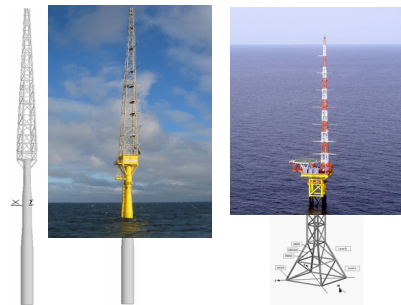
Figure 6: Models and photos of measurement mast Amrumbank West and research platform FINO 1.
